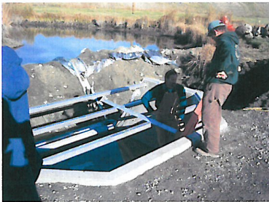
Construction of the fish screen and grating.
