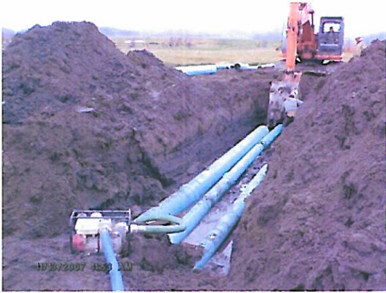
Installation of floodplain/riparian pipelines on the east side of the river November 2007.
