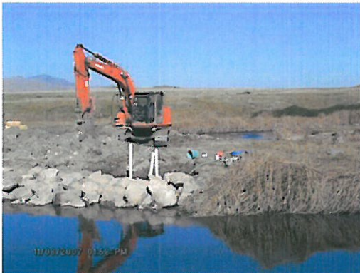
Stream bank armoring upstream from temporary bypass channel inlet (Oct/Nov 2007)
